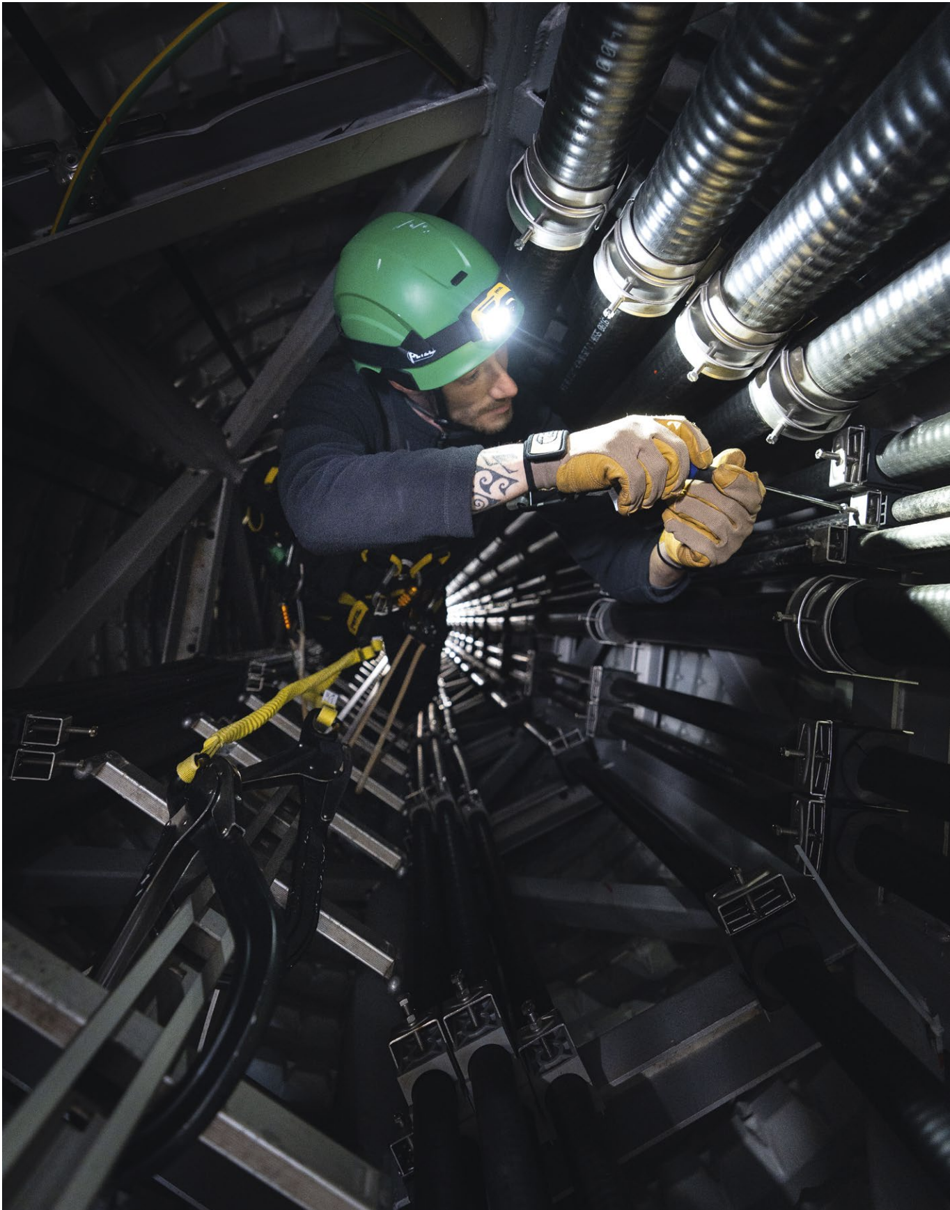
Maintenance operations on a communication tower, Belgium © 2023 Petzl Distribution - Vuedici.org - Monnale
